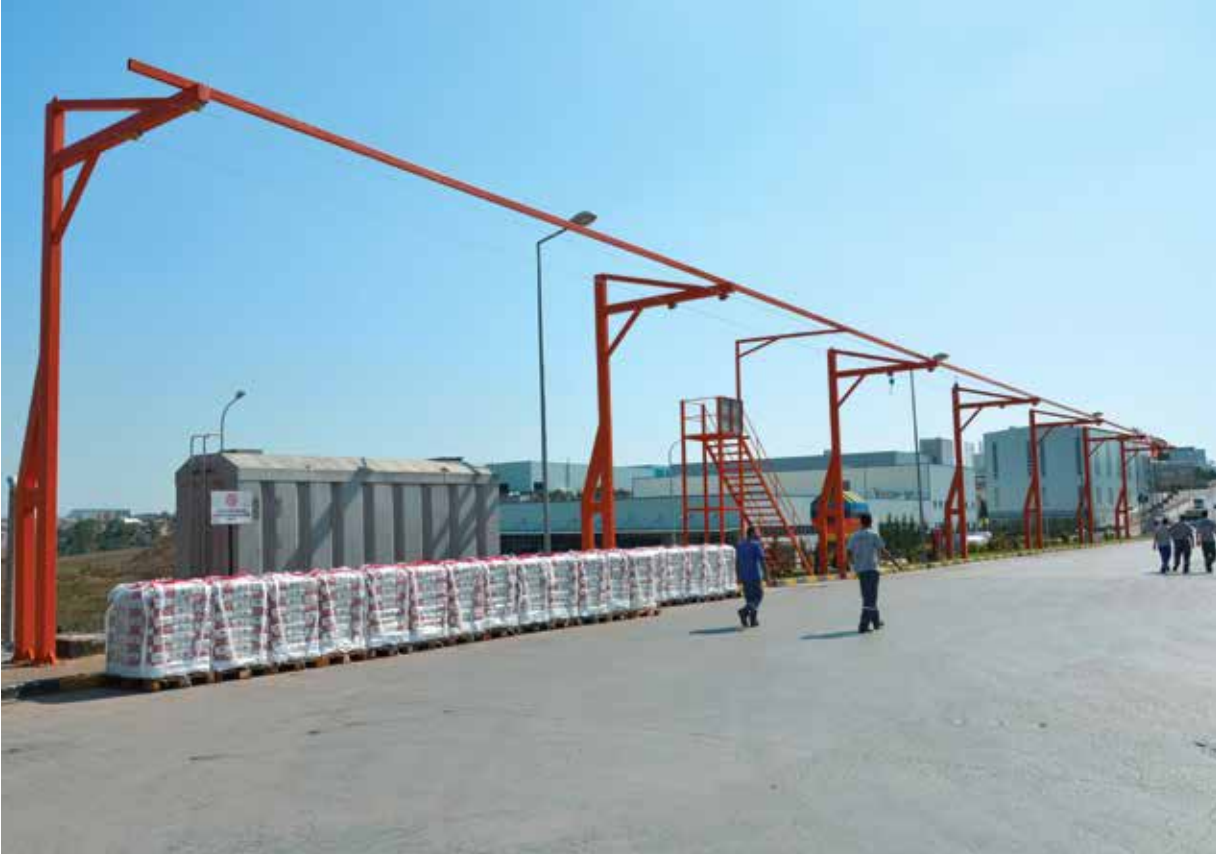
K-2010 HORIZONTAL LIFELINE SYSTEM- TRUCK LOADING & UNLOADING
