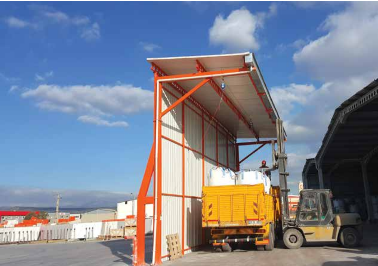
K-2010 HORIZONTAL LIFELINE SYSTEM- TRUCK LOADING & UNLOADING
