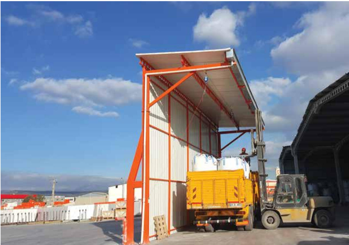
K-2010 HORIZONTAL LIFELINE SYSTEM- TRUCK LOADING & UNLOADING
