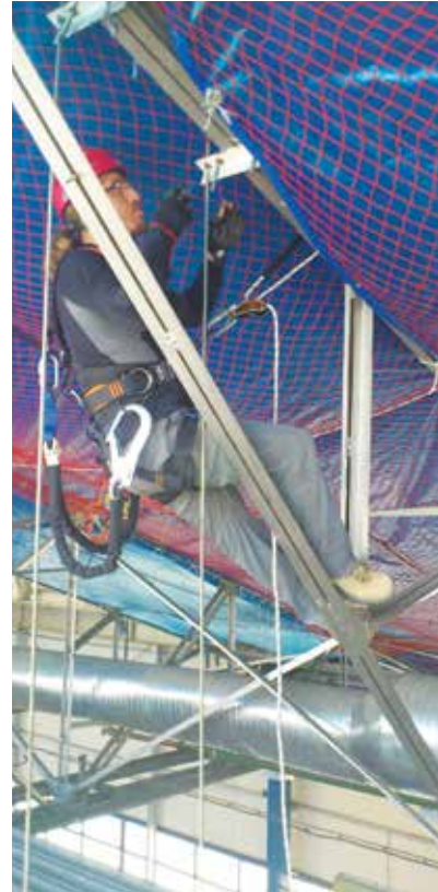
SAFETY NET APPLICATION FOR ROOF CHANGING AT FACTORY
