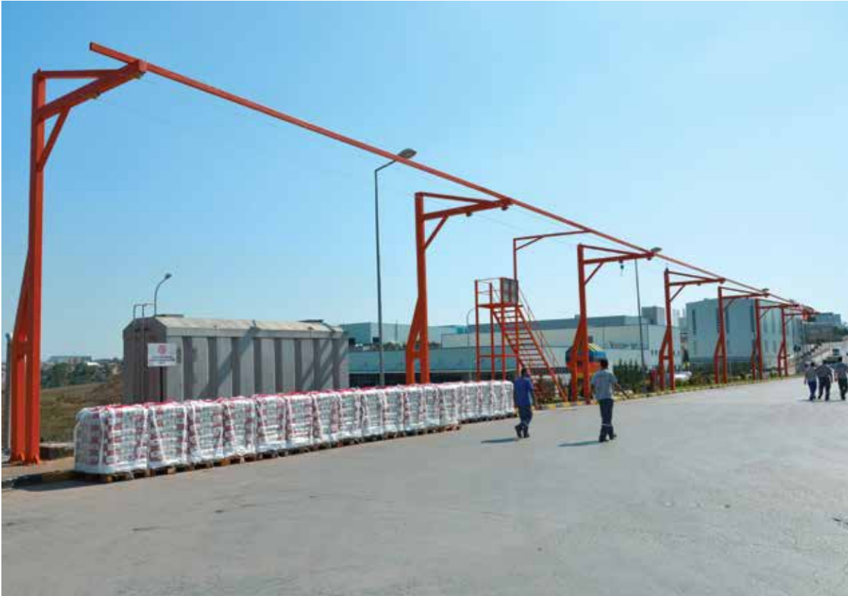
K-2010 HORIZONTAL LIFELINE SYSTEM- TRUCK LOADING & UNLOADING
