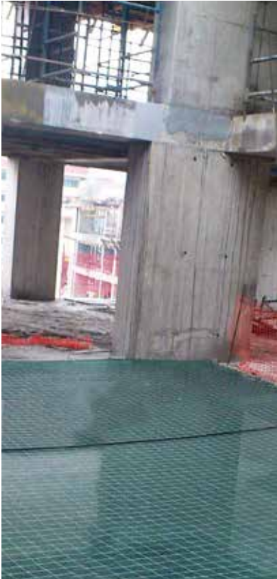
SAFETY NET APPLICATION FOR WIDE FLOOR OPENINGS
