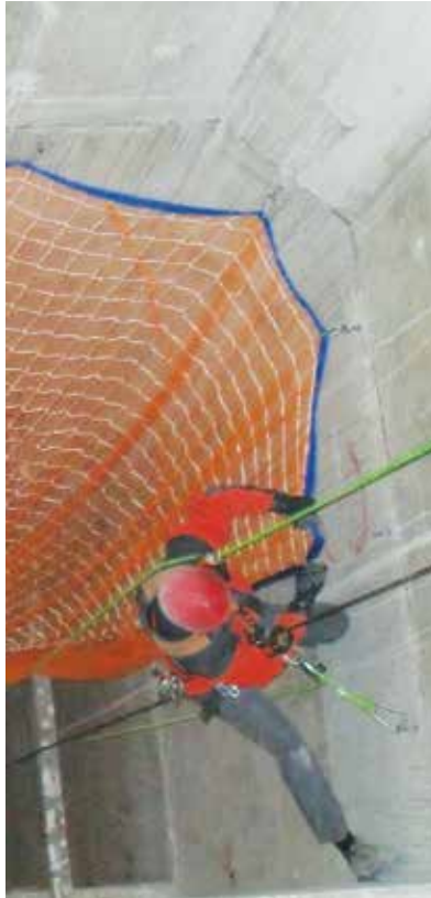
SAFETY NET APPLICATION FOR ELEVATOR SHAFT
