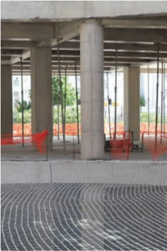
SAFETY NET APPLICATION FOR WIDE FLOOR OPENINGS
