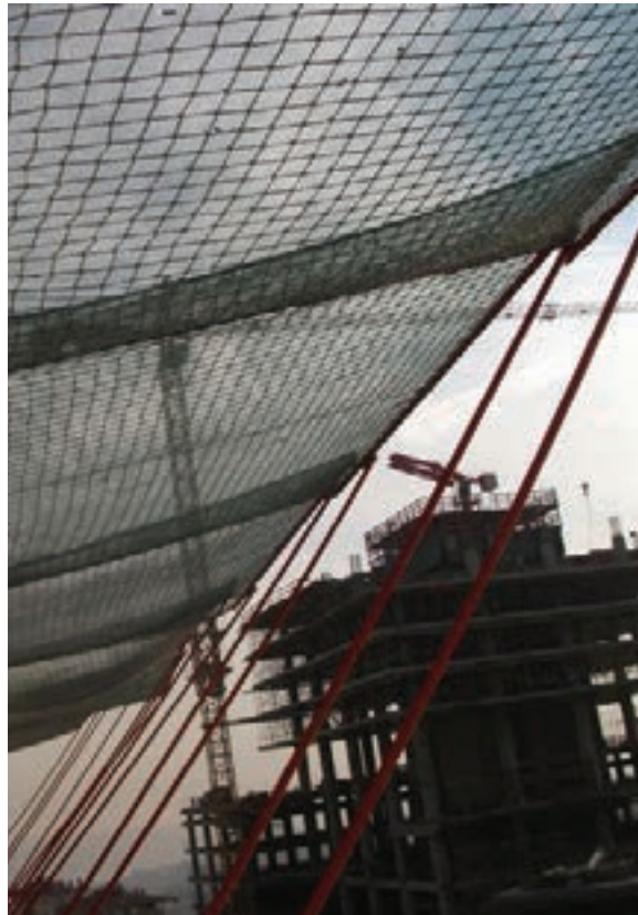
SAFETY NET APPLICATION FOR BUILDING ENTRANCES
