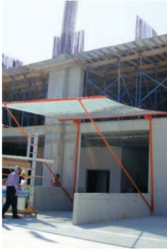
SAFETY NET APPLICATION FOR BUILDING ENTRANCES
