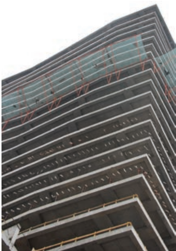
SAFETY NET PLATFORM APPLICATIONS FOR FACADES
