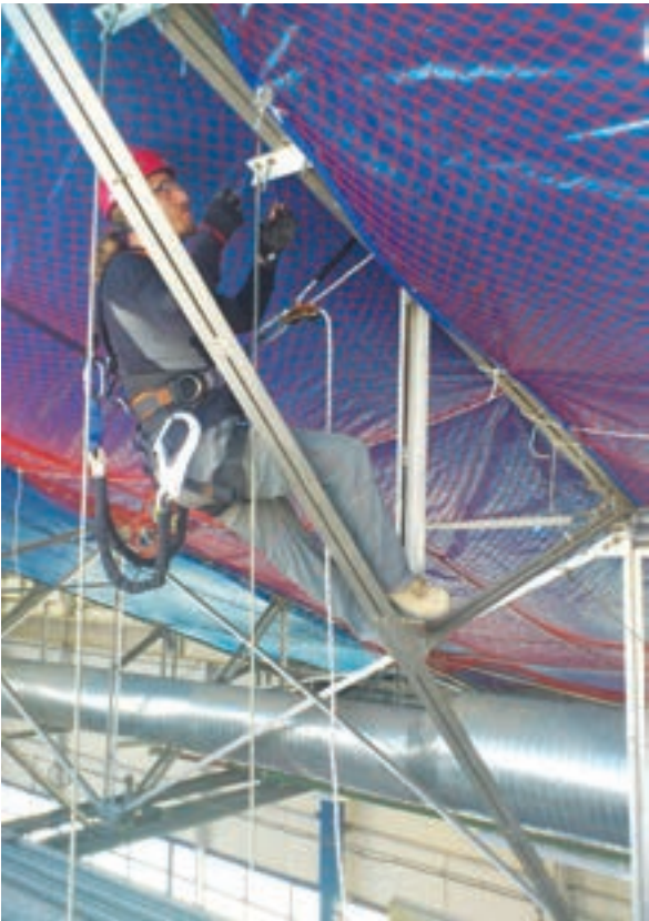
SAFETY NET APPLICATION FOR ROOF CHANGING AT FACTORY
