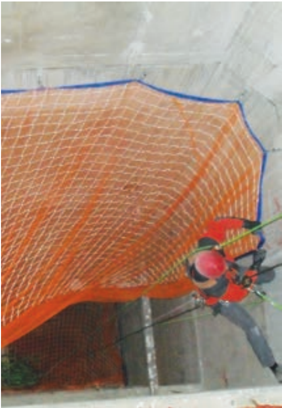
SAFETY NET APPLICATION FOR ELEVATOR SHAFT
