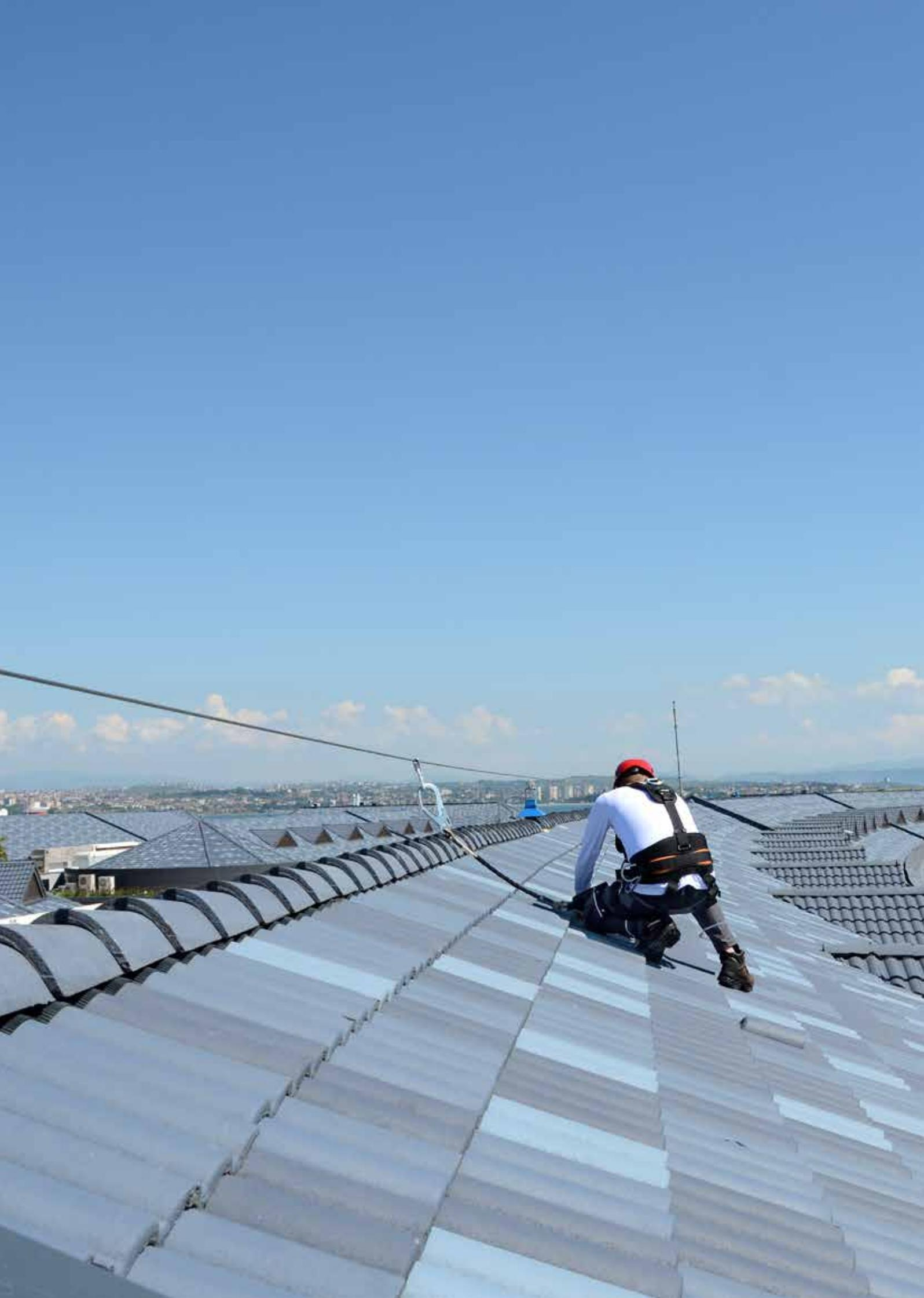
**WORKING ON THE ROOF WITH FIXED HORIZONTAL LIFELINE**
